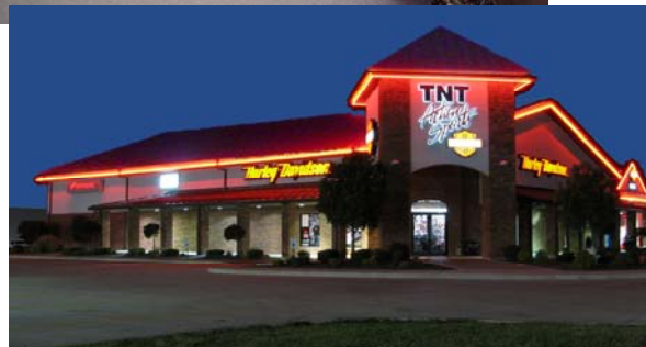
Photos (top to bottom): Ralls County Courthouse mechanical room; Blessing Child Care Facility mechanical room; TNT Harley Davidson facility exterior lighting.
